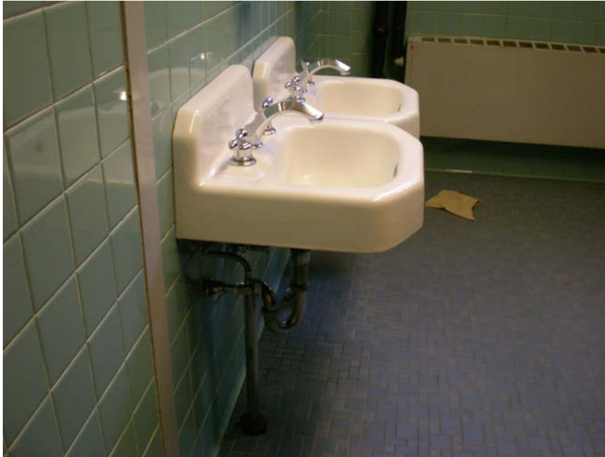
Lavatories at BOYS TOILET 52
